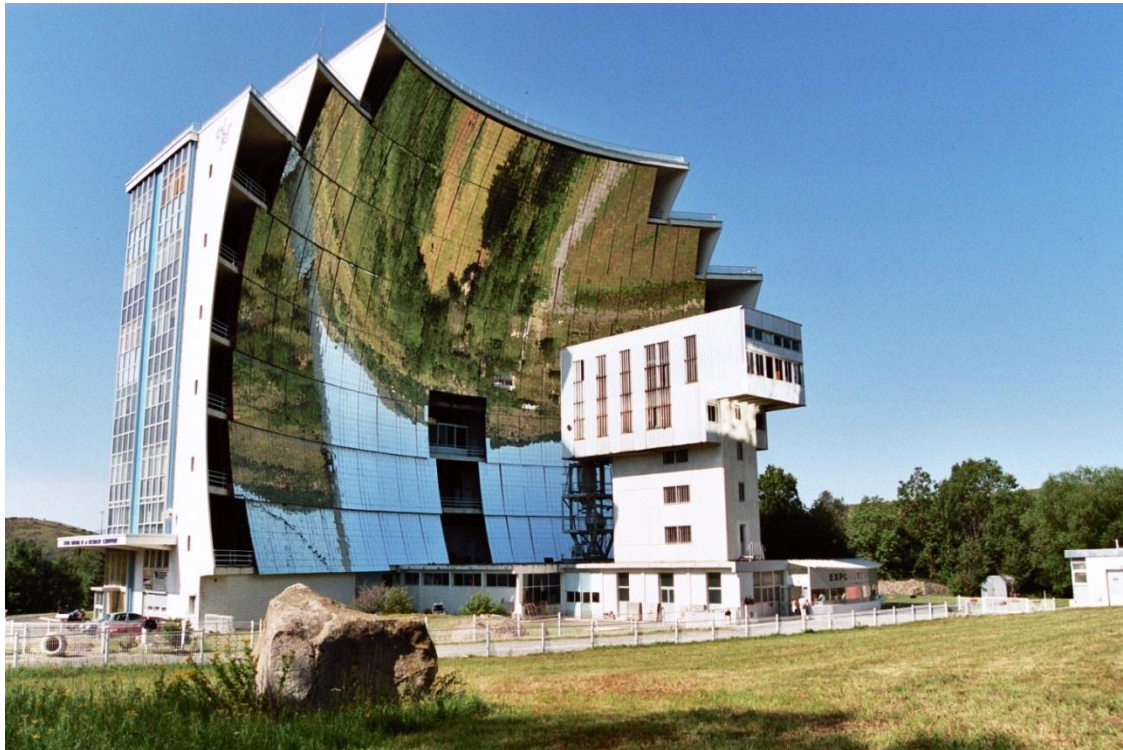
Figure 2.5 View of the world's largest solar furnace at Odeillo in Pyrenees-Orientales France[1].
